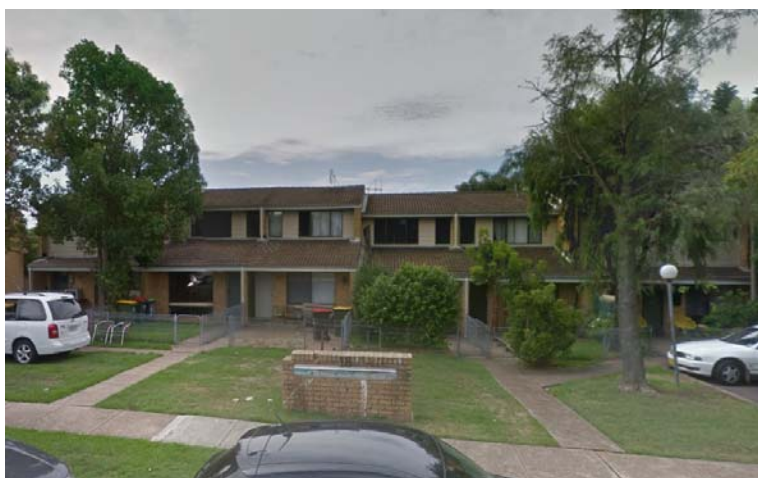
Photograph 5: Medium density residential development adjacent on Tinonee Road, Waratah.
