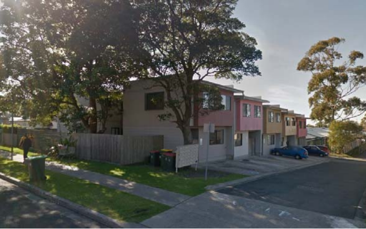
Photograph 1: Existing 5 student accommodation townhouses, corner 58 Harriet Street, Waratah.
